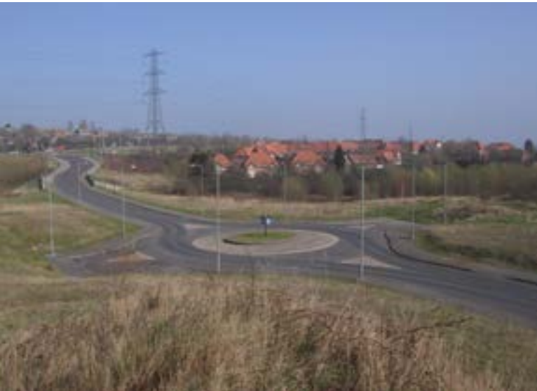
Existing road infrastructure
