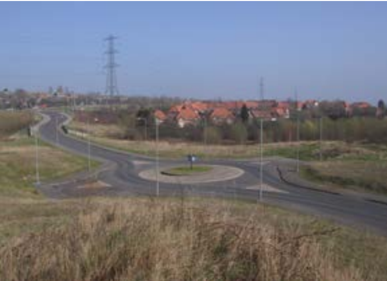
Existing road infrastructure
